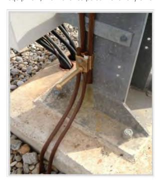
DSA Copperweld \* wire and strand have the high current-carrying capacity characteristics in short-time durations, high strength properties and corrosion resistance to effectively and economically meet IEEE recommendations. These advantages are particularly evident when compared to a low-strength material such as solid copper. Solid copper conductors must be upsized in many installations to meet the mechanical demands within a system design.
